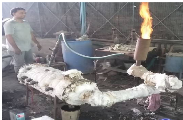
Fig. 2. Horizontal gasifier in operation after insulation
